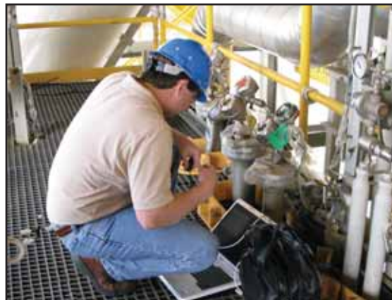
An Orion technician operates PACTware on a drilling rig
