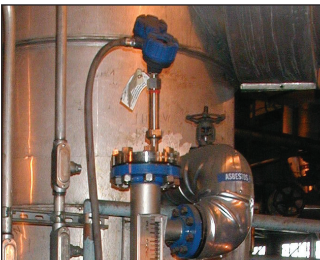
GUIDED WAVE RADAR UNITS OFFER MORE ACCURACY IN HARSH ENVIRONMENTS.
